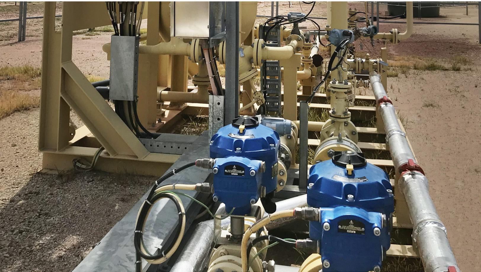
The Rotork CVQ electric actuators will operate ball and v-ball valves on separator skids at an Australian onshore natural gas production site.
